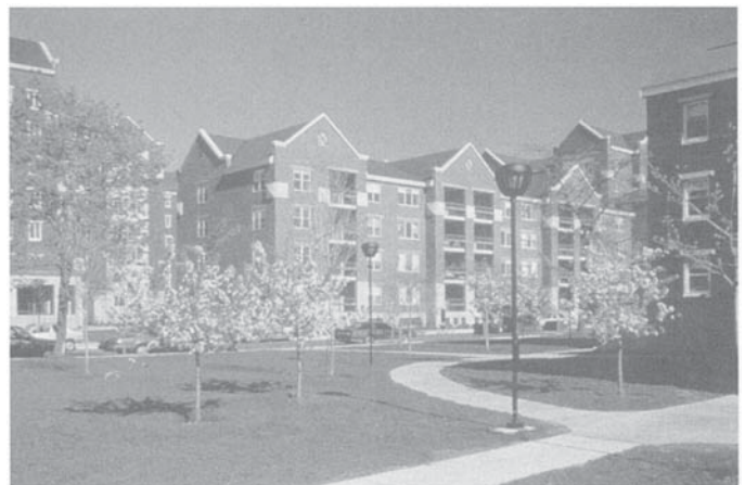
Fig. 10. The adaptive re-use of public housing into a mixed race and income community at Harbor Point models a move from 20% occupancy in Columbia Point to 98% in the Harbor Point of 1996 and a shift from 100% low income in Columbia Point to 70% market rate and 30% subsidized low income units.
